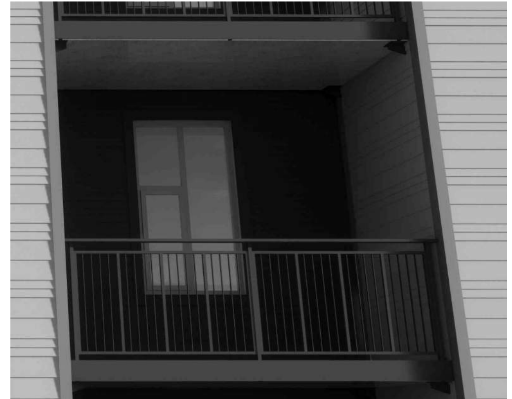
Metal Railings - Face Fastened to Wood Frame Balconies
